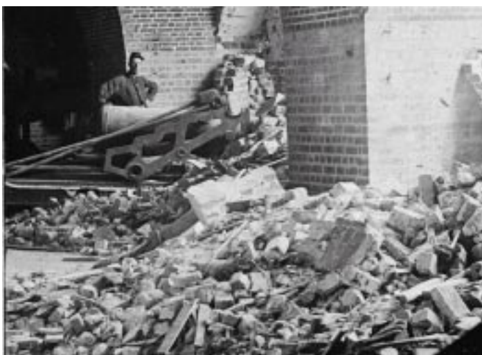
Casemate damage in the interior of Fort Pulaski after the bombardment. Brick could not withstand rifled cannon.
