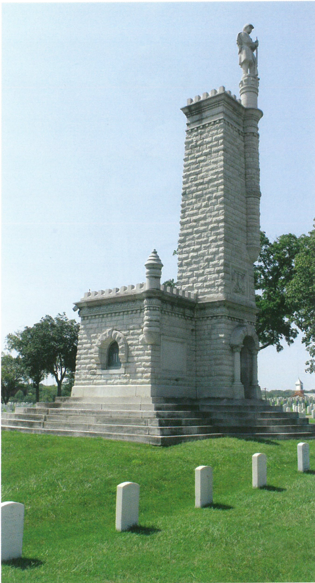
The Tennessee Grand Army of the Republic monument, Knoxville National Cemetery. The cornerstone of the monument states “In Memoriam Union Soldiers of Tennessee October 15, 1896.” Originally topped with an eagle, the monument was struck by lightning in 1904. It was rebuilt and rededicated in 1906 with the figure of a soldier replacing the eagle. Author’s collection.
